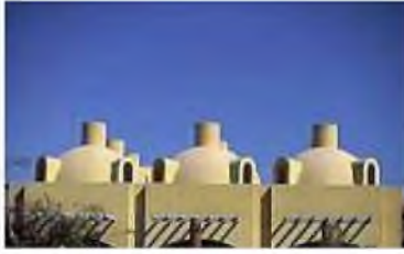
Miramar Resort Hotel - arcspac.com arcspac.com
