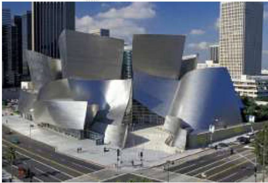
Walt Disney Concert Hall (Los Angeles, U.S., 2003) | IMAGE COURTESY OF GEHRY PARTNERS, LLP
