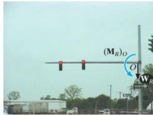
The weights of these traffic lights can be replaced by their equivalent resultant force  $W_R = W_1 + W_2$  and a couple moment  $(M_R)_O = W_1 d_1 + W_2 d_2$  at the support,  $O$ . In both cases the support must provide the same resistance to translation and rotation in order to keep the member in the horizontal position.
