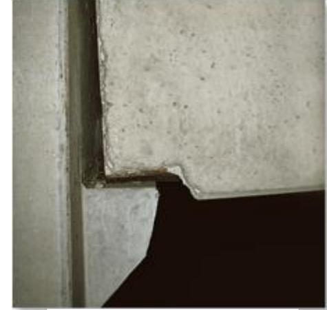
This concrete girder rests on the ledge that is assumed to act as a smooth contacting surface. (5)
