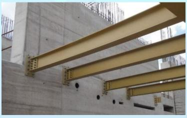
The same situation appears in the case of a clamped support (fixed support) according to figure b which symbolically is depicted in figure c. The free-body diagram in figure d shows that the clamped support can transmit a reaction force A of arbitrary magnitude & direction (or  $A_H$  and  $A_V$ ) and a couple moment  $M_A$  (or  $A_M$ ).
