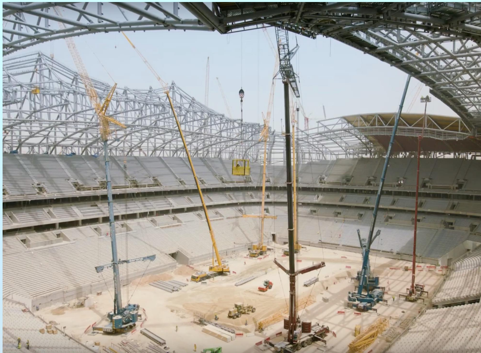
Construction of one of World cup stadium in Qatar
