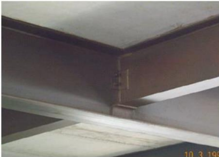
Secondary beam-main beam connection (web cleat) (assumed as pin connection)
