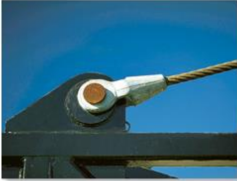
The cable exerts a force on the bracket in the direction of the cable. (1)
