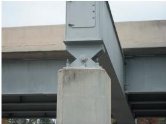
Typical pin support for a beam. (8)
