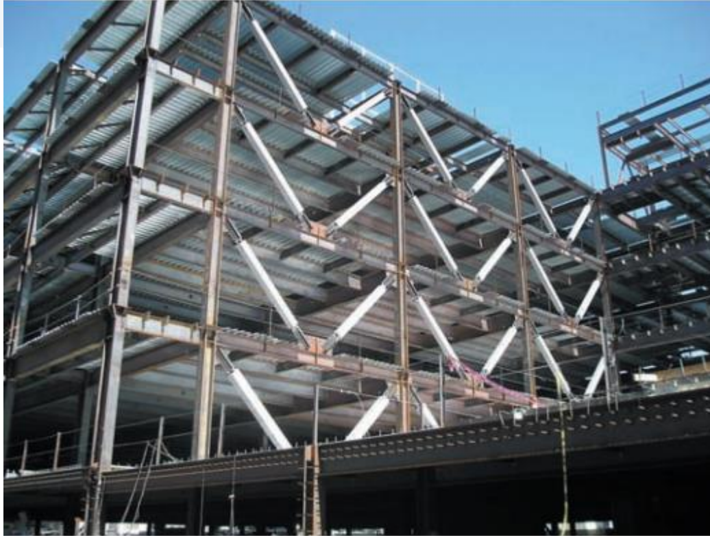
Multistory Building with Braced Frames to Transmit Lateral Loads Due to Wind and Earthquakes
