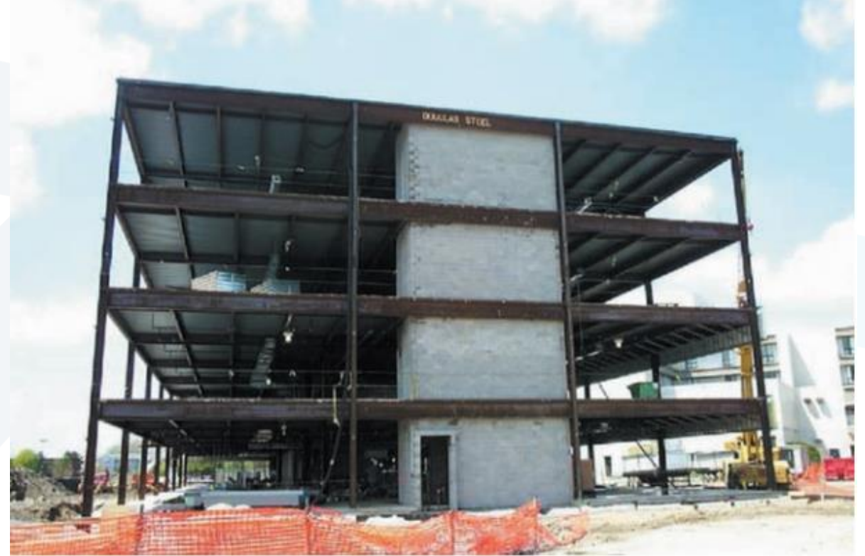
This Steel Frame Building Uses Masonry Shafts for Elevators and Stairs to Resist Lateral Loads Due to Wind and Earthquakes
