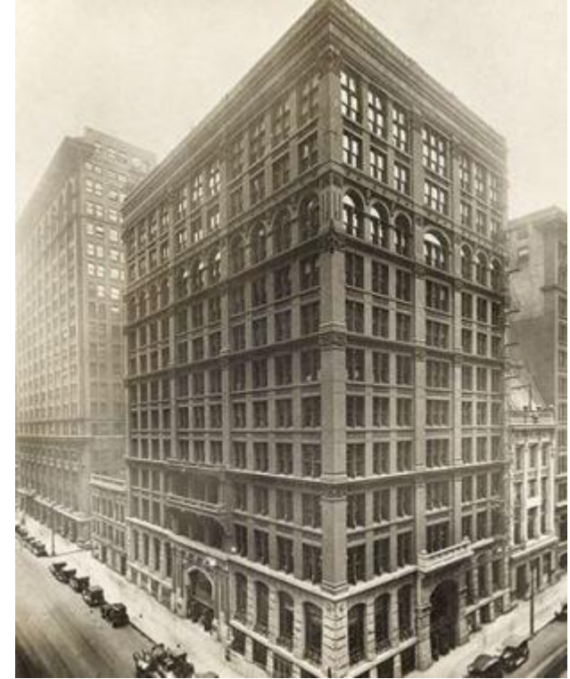
Rigid Frame Systems (Home Insurance Building, Chicago, USA)
