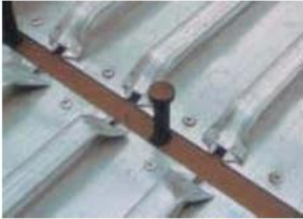
Non continuous metall decking over the beams
