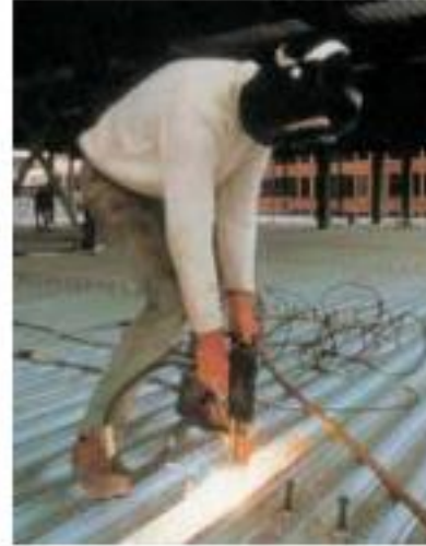
“Through deck welding” on site
